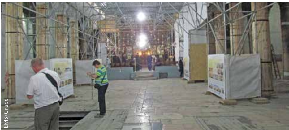
The interior of the Church of the Nativity during restoration work.
