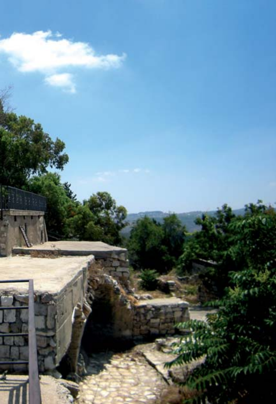
The Maronite church in Bar'am is the only building that has been restored in the village destroyed in 1953.
