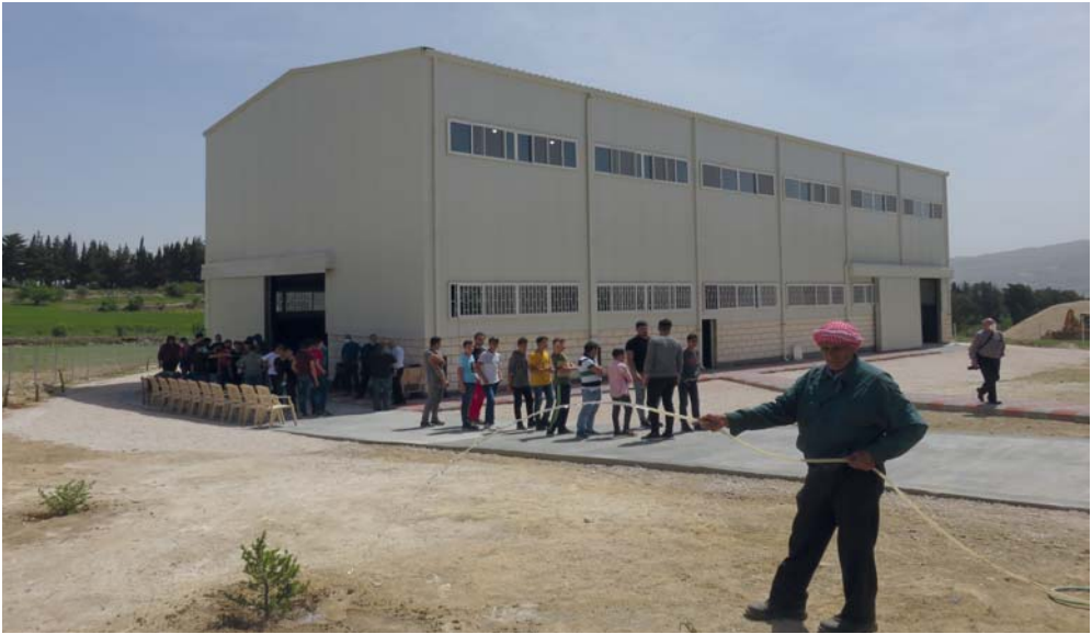
The new carpentry workshop: big, functional and built with an eye to the future.
