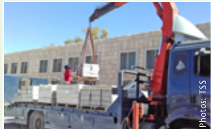
The first modules of the photovoltaic system are lifted onto the roof of the boarding home.
