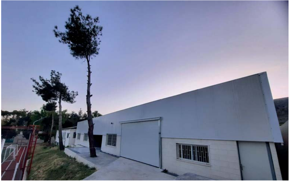
The new hangar where the electrical apprentices have already moved to. In future, this is also where vocational training on electric cars will take place.
