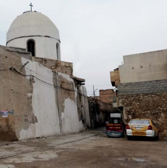
The IS occupied St George's Church in Mosul for three years, smashing all the crosses and destroying the interior. Nothing has been restored yet. An inscription on the outside wall says: "Just as I have loved you, you also should love one another." (John 13:34)
